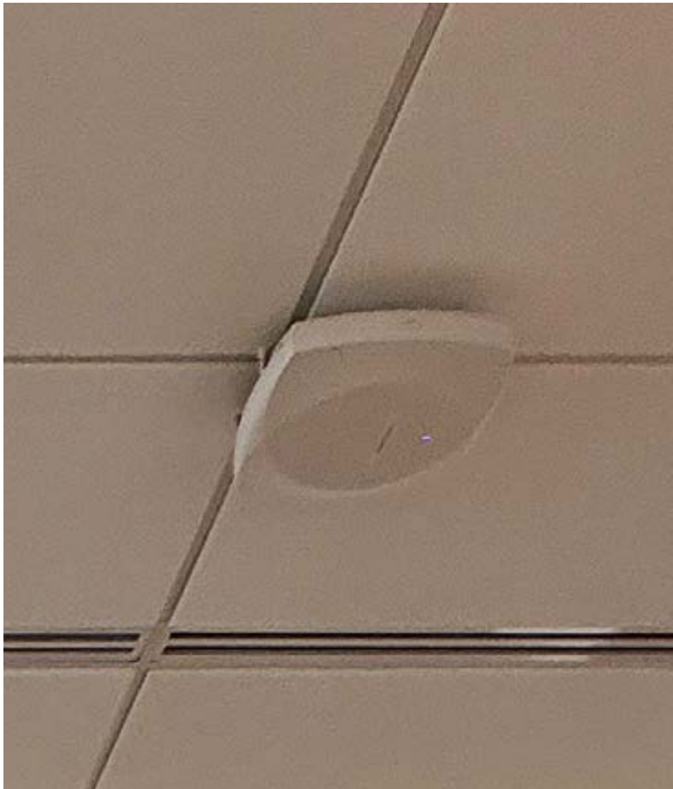
Cisco Wireless 9178i Access Points
